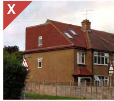
Figure 4.21g: Example of where a highly visible roof extension dominates the original building and negatively impacts the appearance of the street. This could have been avoided had the rear box extension been set in from the gable end of the roof to allow the gable and the rear extension to read as two separate elements.
