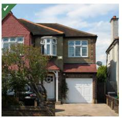
Figure 4.17a: A good example of a setback at first floor on a two-storey side extension.
