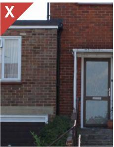
Figure 4.26b: An example of a side extension that attempts to match the existing brick work but fails to do so.
