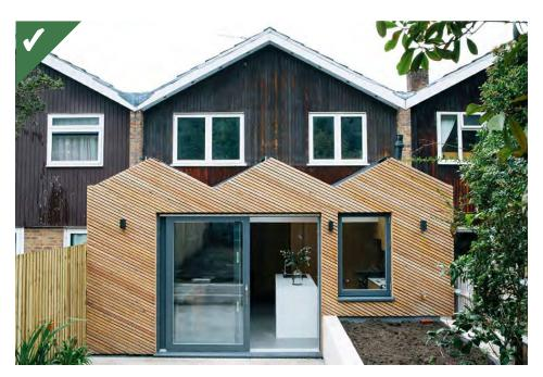
Figure 4.15a: An example of a roof design to a single storey extension by Nimtim Architcts that has been designed to ensure it doesn't overlap with the windows above. (Photo: Anna + Tam)
